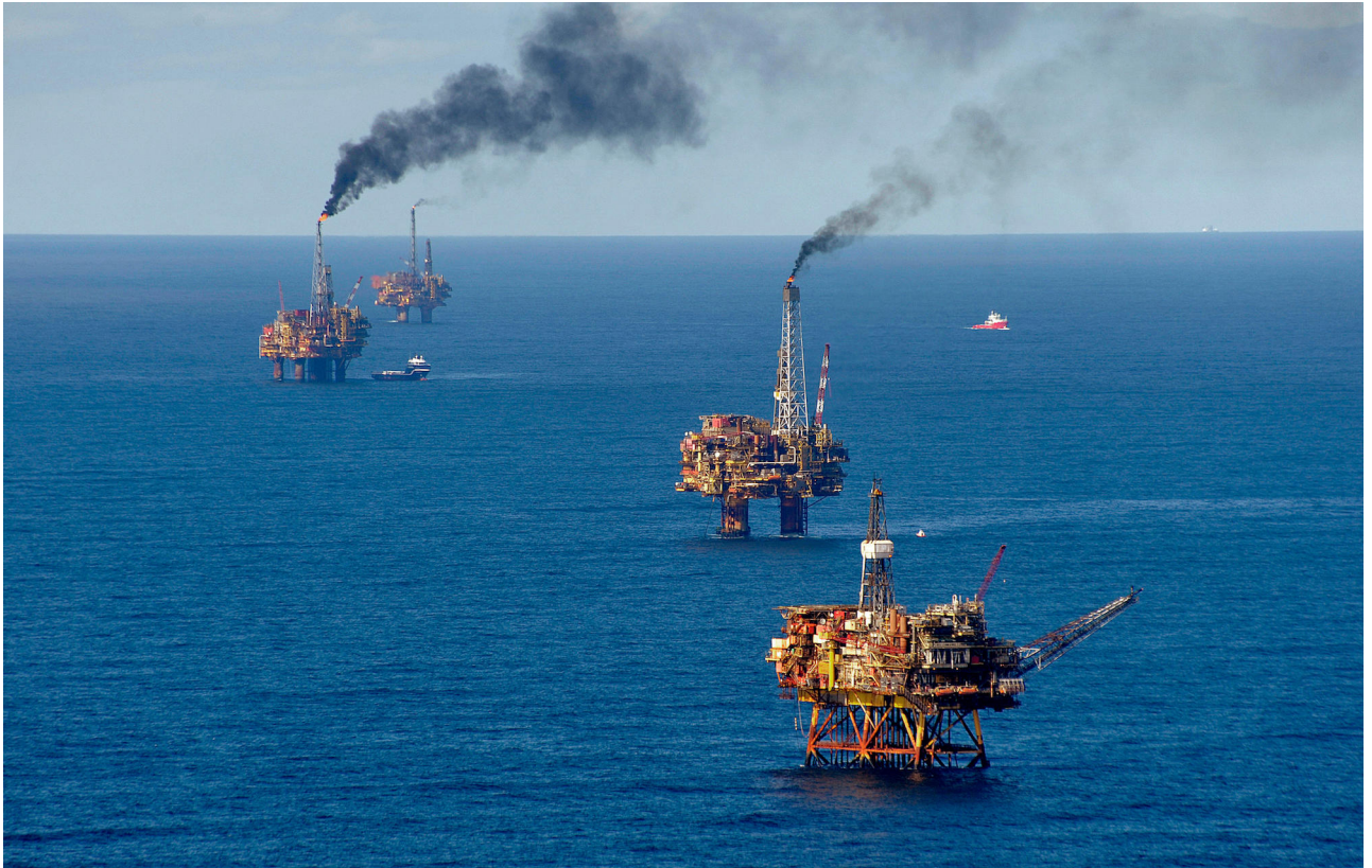
KRT18T North Sea, Oil production with platforms. Aerial view. Brent Oil Field.
